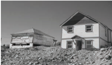
One of the two unfinished Victorians stands next to one of the two finished Victorians on Porphry St
